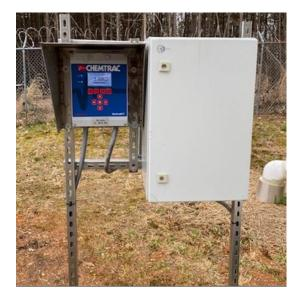
Chemtrac chlorine analyzer remote installation next to distribution system water storage tank.
