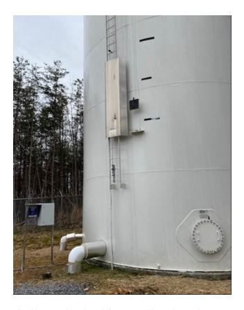
The chlorine analyzer (lower left) is powered by a solar panel located on the top of the tank.
